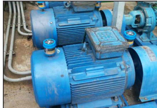
A combination of high-performance grease applied in a controlled manner via the Chesterton Lubri-Cup.
